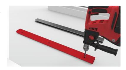
c) Fasten the guide to the window frame using a self-drilling screw.
