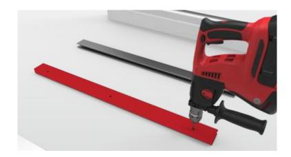
b) Deepen the holes made to the depth of the first wall of the guide (its thickness) with a  $\emptyset$  10 mm drill.
