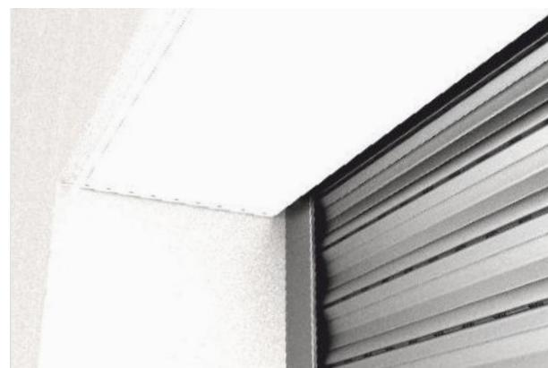
EN | stiff, aesthetical and functional design of the bottom profile and access plate (revision of the entire depth of the box)
