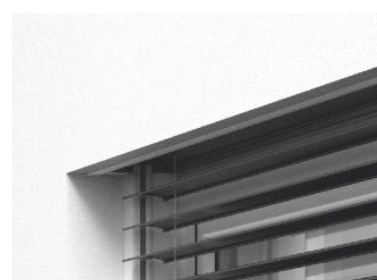
architectural cleanliness due to the fully covered box
